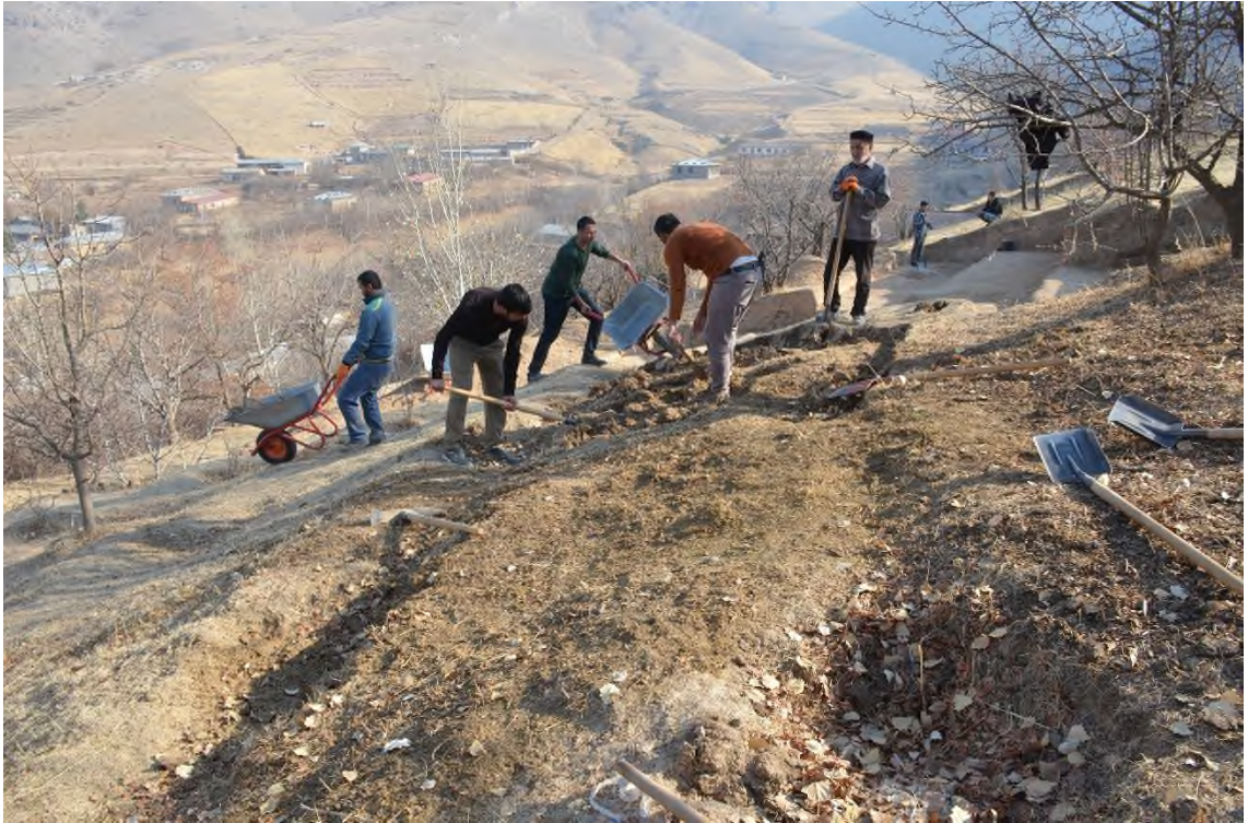
Figure 8 – Opening of the upper layer (Excavation 4). Work in progress.
