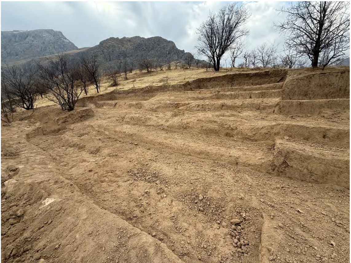
Figure 88 – General view after reclamation
