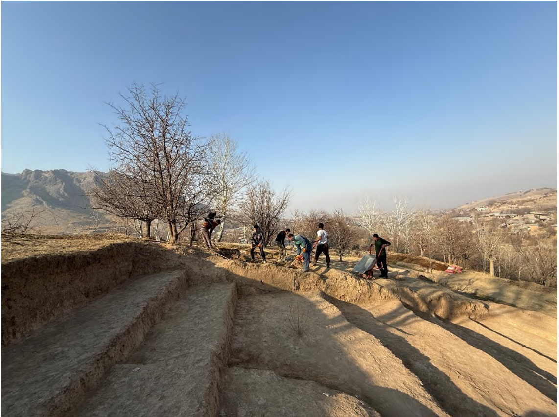
Figure 6 – General view of the excavation prior to the commencement of works (Excavation 4). View to the northwest.
