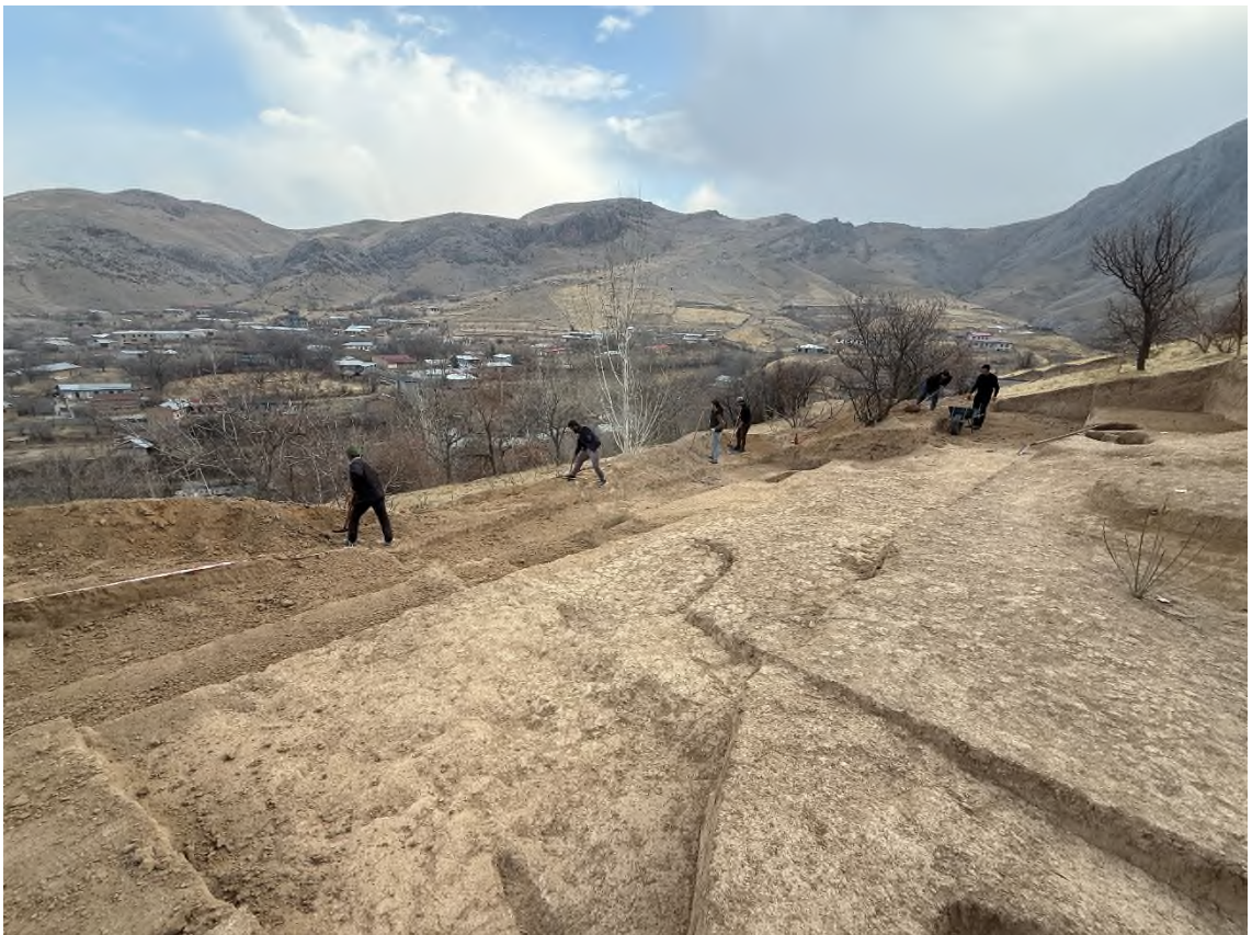
Figure 87 – Process of excavation reclamation
