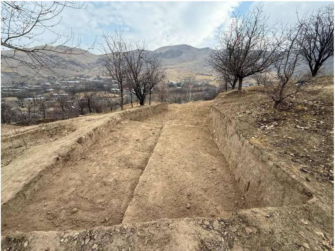
Figure 90 – General view after reclamation
