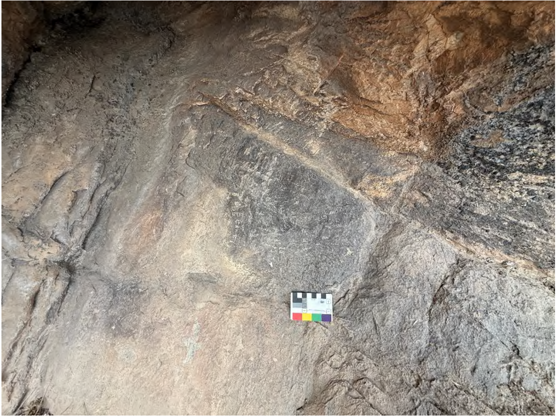
Figure 5 – Upper platform (grotto). Lower surface of the grotto
