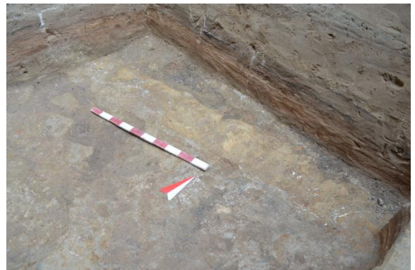
Figure A.196 - Element 109, 110. Masonry of the wall made of fine-grained raw sanded yellow bricks and a layer of laid broken raw bricks. View to the northwest.
