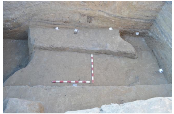
Figure A.68 - Elements 87, 88, 89, 90, 91, 92. General view of the trench after removing the layer of dense bright brown loam with charcoal inclusions (92). View to the south.
