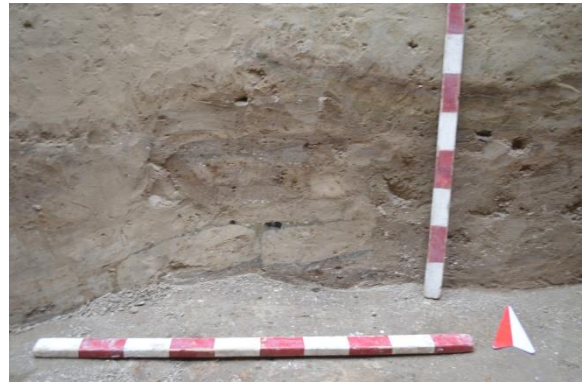
Figure A.46 - Element 85. Brickwork in the cross-section of the wall (94) after excavating the fill layer inside the garbage pit (ditch). View to the north.
