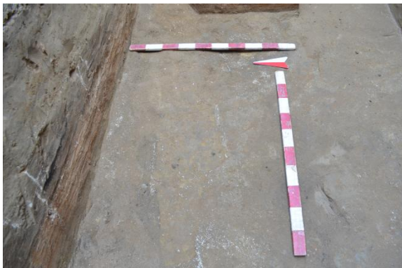
Figure A.195 - Element 109, 110. Masonry of the wall made of fine-grained raw sanded yellow bricks and a layer of laid broken raw bricks. View to the east.
